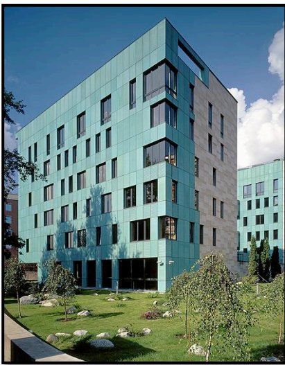
S.Skuratov, Copper House, 2005
