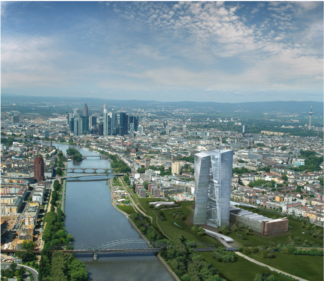
The New ECB Premises (on the site of the former Grossmarkthalle) with Frankfurt's financial district in the background; view from the east.
